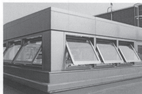
Ventilation windows on the roof
